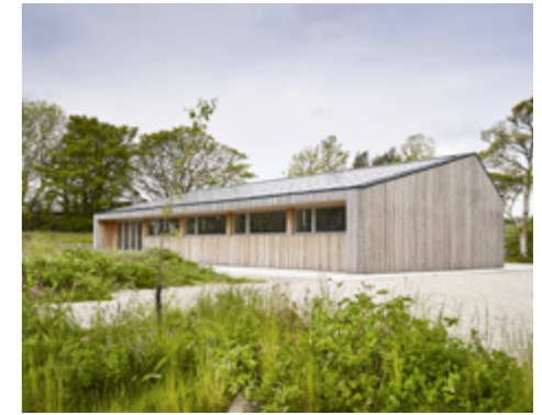
Argal Workshops (Gluckman Smith) A Cornish former farmstead, previously derelict, was transformed into rural workshops for a local furniture and product designer, to Passivhaus standards, making a new working community for the area.
