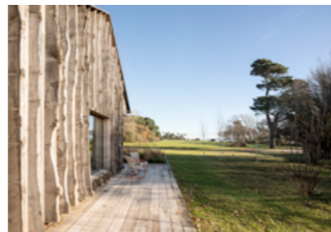
The Barn by Pad Studio Planks of wood reclaimed from an old barn were used to clad this house in Hampshire, England, designed by Pad Studio.
