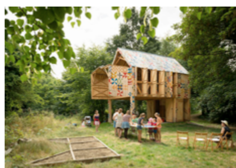
Ecology of Colour, Dartford by Studio Weave Part of a project to bring public function and engagement with local ecology to a neglected corner of Dartford.
