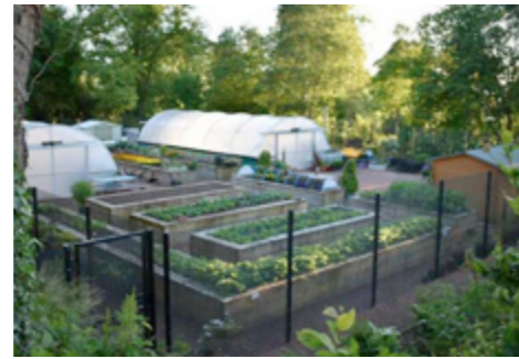
Castlebank Horticultural Training Centre, Lanark (EKJN) A collection of neglected outbuildings have become a thriving horticultural training centre, a valuable community resource.
